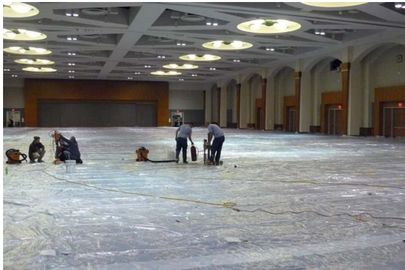
Above: CRC crews work to core drill strategically-placed grouting injection holes within the main ballroom areas of the Frontier Airlines Center. Plastic sheeting appears over the carpeted ballroom floor. Flaps were cut in the carpet for grout injection holes.
