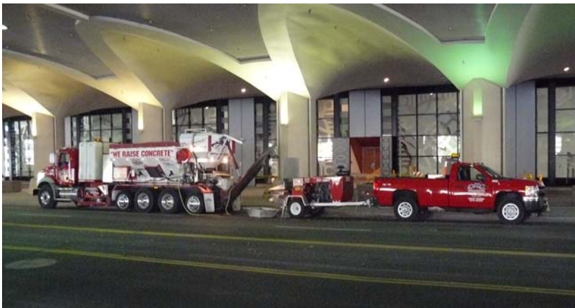
Above: A CRC volumetric mixer is shown producing fresh grout at the Frontier Airlines Center. The grout was being mixed into a 60-yard concrete pump (shown at the back of the work truck) and pumped to the interior ballroom, where the line was reduced and the material injected.
