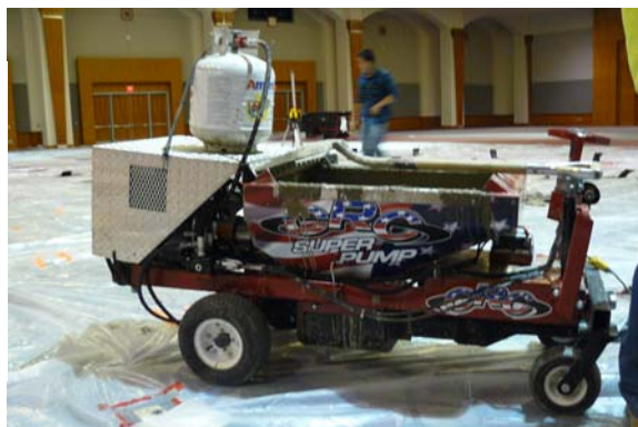
Above: A CRC volumetric mixer is shown producing fresh grout at the Frontier Airlines Center. The grout was being mixed into a 60-yard concrete pump (shown at the back of the work truck) and pumped to the interior ballroom, where the line was reduced and the material injected.
